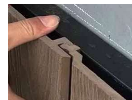
Step 6 Install the rest of the wall panels into the first wall panel.
