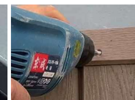
Step 7 Drive screws on top of the side cover
