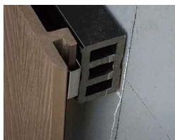
Step 5 Slip the first wall panel against the starter clip firmly.
