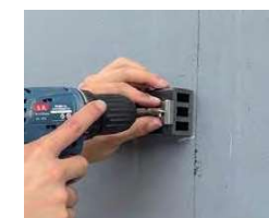
Step 4 Set a starter clip at the end of each joist with a stainless steel screw.
